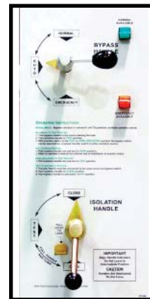
Bypass and Isolation Operating Handles
